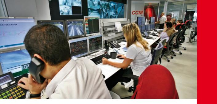
The CCM operates 24 hours a day, all year round, ensuring that the programmed service is provided with maximum quality. This means controlling the regulation of intervals between trains, adjusting supply to suit demand in real time, managing night work and the internal and external information channels, and drawing up studies on the service. It also deals with unforeseen events, coordinating action to resolve any incidents or emergencies that may arise.
